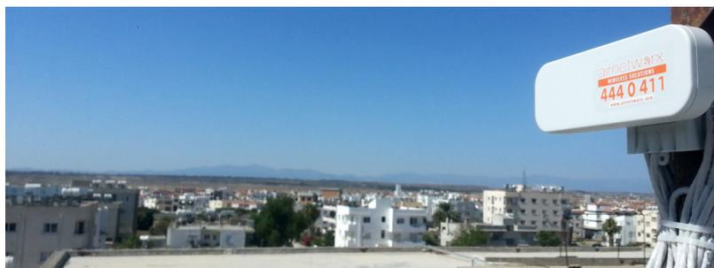
**LigoPTP UNITY 5-N** devices were selected for the backbone of the network, which did a perfect job ensuring the minimum required capacity of 130 Mbps without any disturbance.
